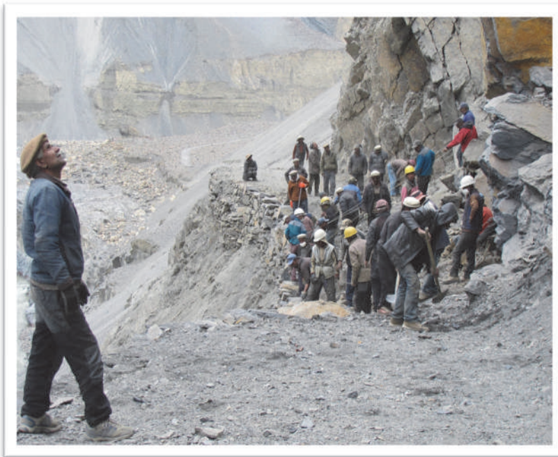
Figure 2: Shimshal Community Volunteers Repairing Blocked Road, Veyeenben Shimshal
