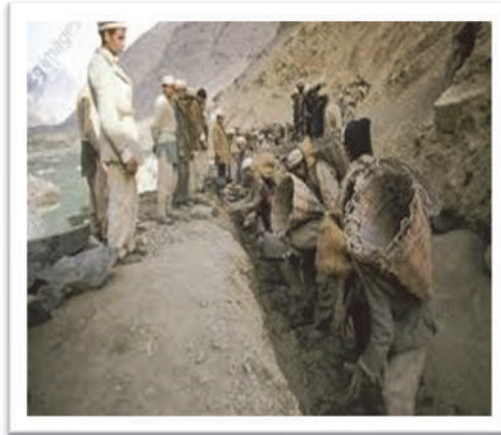
Figure 6: Constructing Water Channel with No External or Government Support
